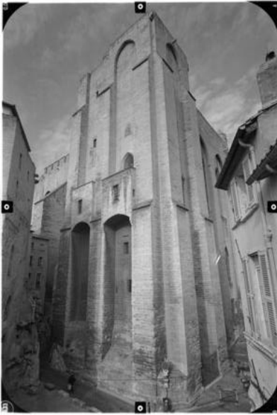
Tour Saint-Laurent south-east overview
